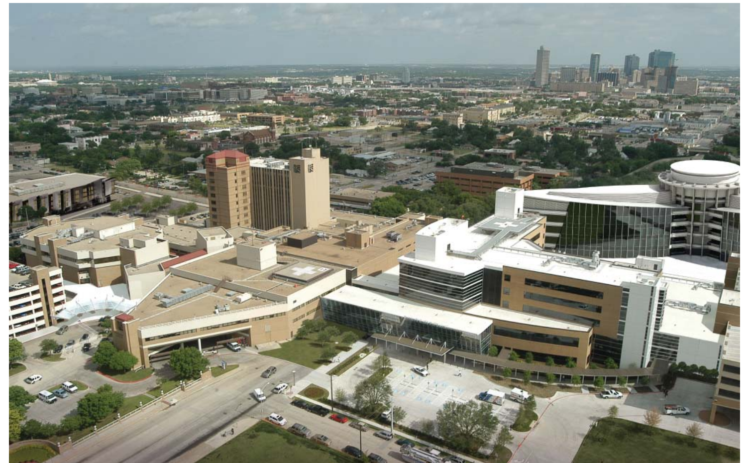
Proposed New Inpatient Bed Tower and connection to adjoining existing JPS hospital
