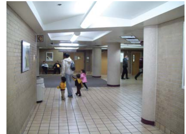
Lobby area, limited visibility to elevators
