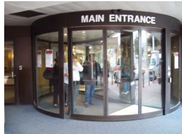
Main Entrance Revolving Door
