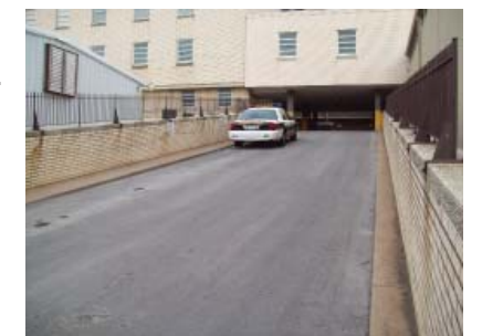
Police Entrance Ramp
