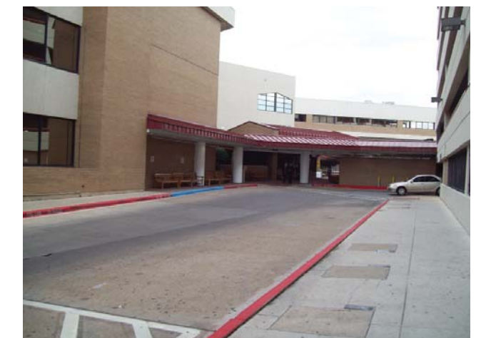
Street/walkway between front entry and main parking garage.
