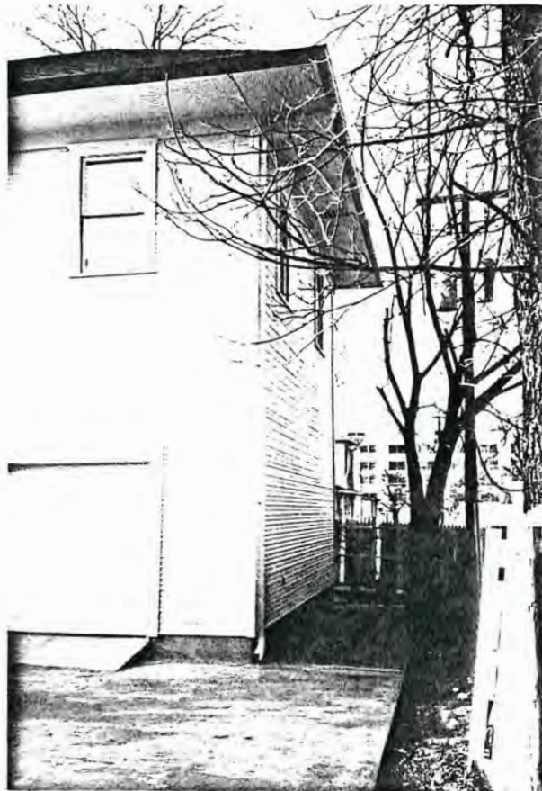
Back of House facing East
