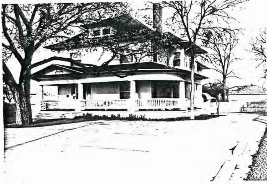
Front of House faces West
