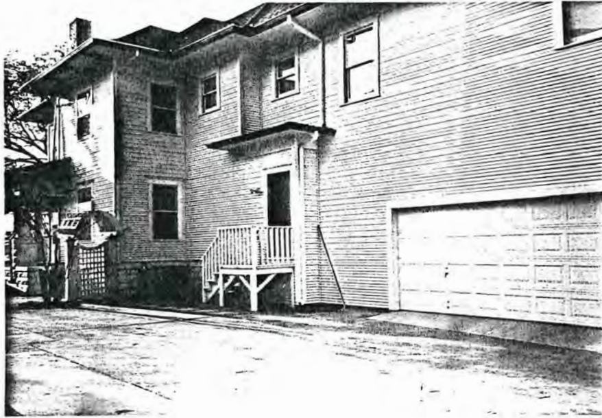
South Side of House
