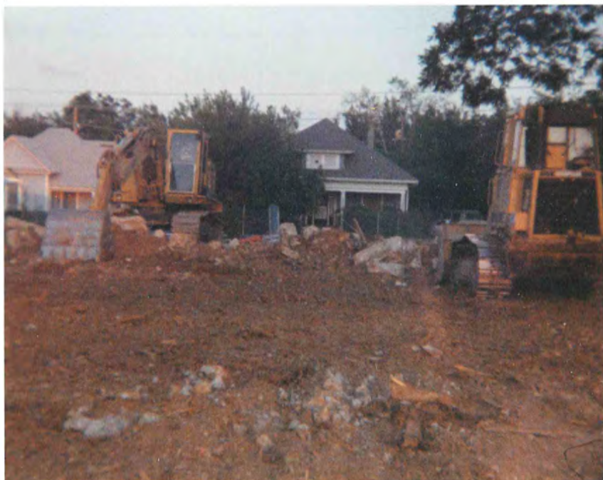
1993 Demolition Just to the North of the House
