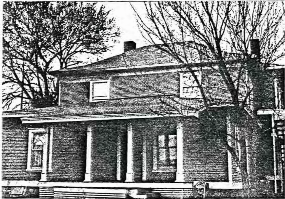
A small enclosed porch was removed from the back of the house where the addition was added. The same type of roof line was kept to match the original structure.
