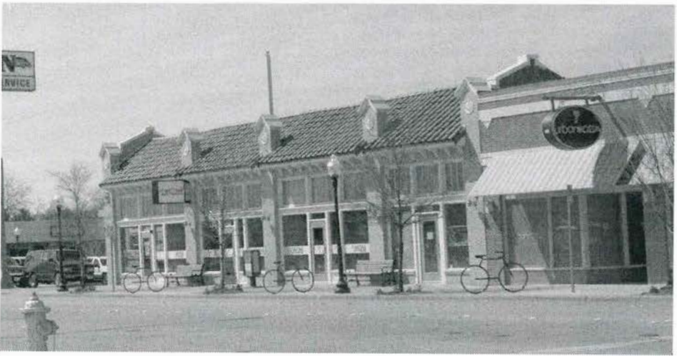
Figure 3: Comparative property in 1700 block 8 th Avenue. One-part Commercial Block with multiple storefronts. The brick is painted.
