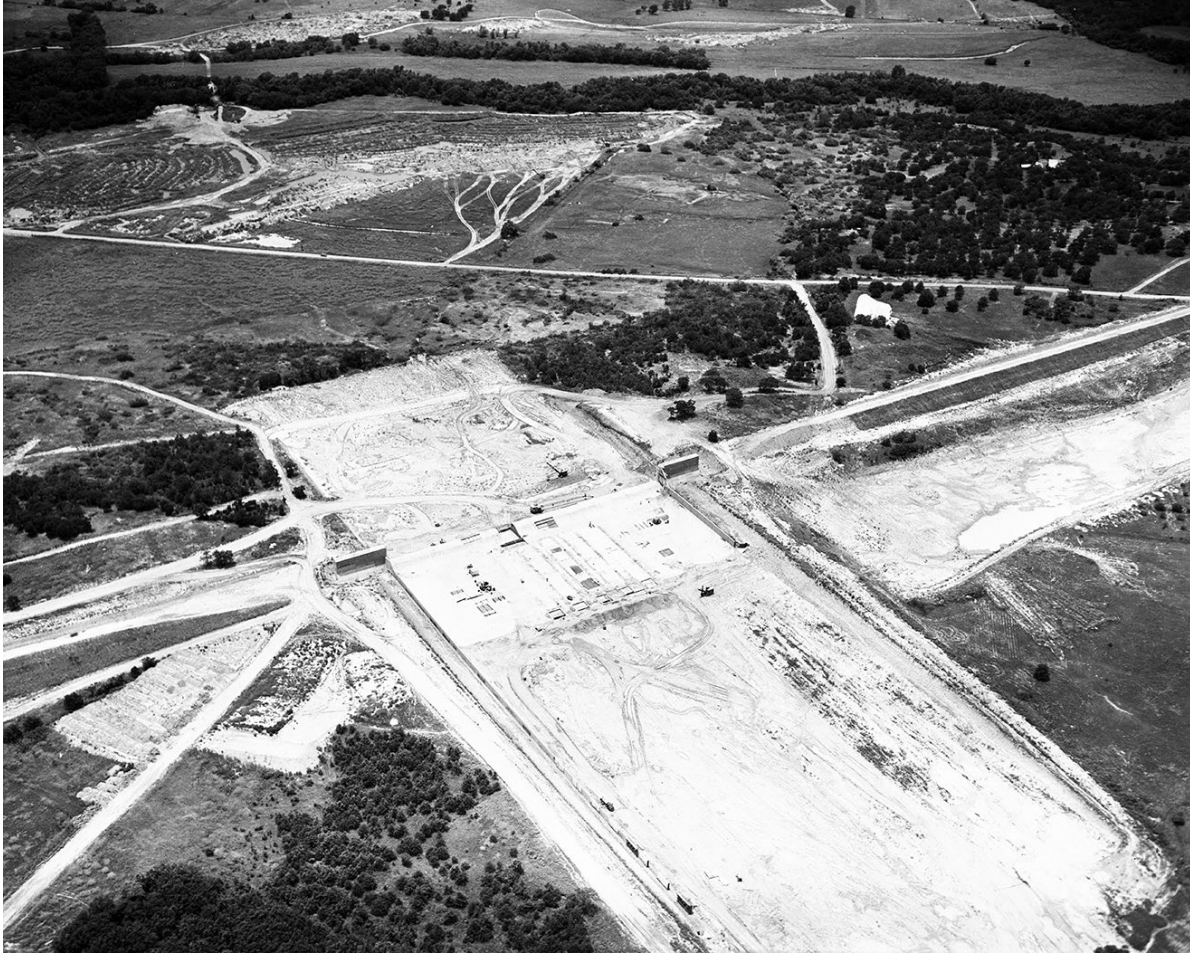
Figure 6-5. Aerial view of the construction of Grapevine Dam in 1950. Parts of the dam that are visible include the concrete spillway, concrete tie-ins to the earthen embankment, and the spillway channel with a retaining wall. Source: Fort Worth Star-Telegram Collection, University of Texas at Arlington Libraries. "Aerial view of the Grapevine spillway." UTA Libraries Digital Gallery, 1950, Accessed June 5, 2024, https://library.uta.edu/digitalgallery/img/20148066 .
