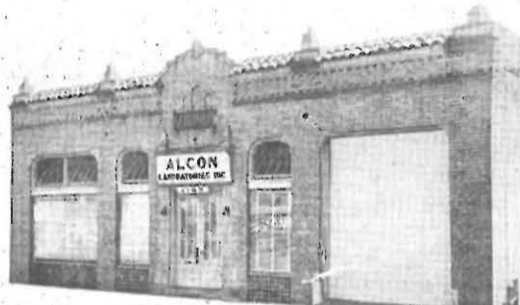
An undated photo of an early Alcon facility. The company is celebrating its 50th anniversary.
