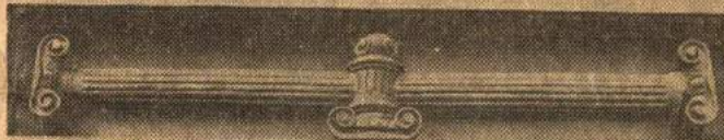
DOORWAY DETAIL —Column treatment over front doors both inside and out is formed of wooden decorations which once were part of a horse-drawn hearse.
