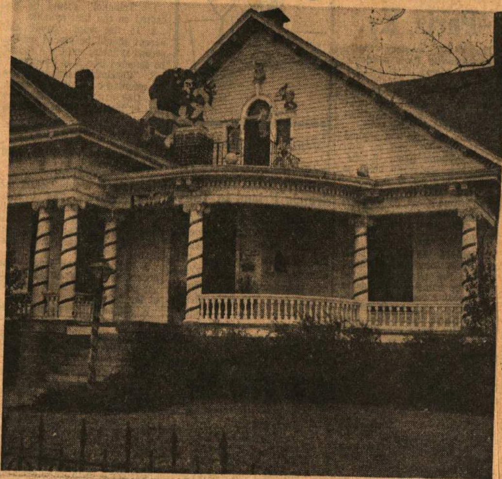
LANDMARK—The former home of the late Mr. and Mrs. John Jacob Reimers at 428 S. Adams, now being demolished, is shown in its holiday trimmings when the last owners, Mr. and Mrs. Lester Moss, lived there.
