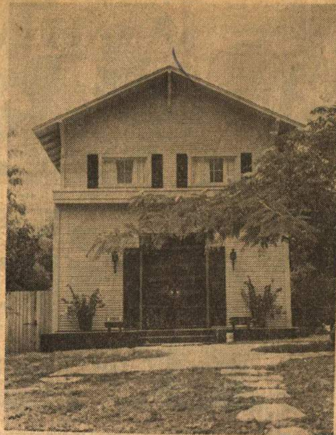
IMPROVED VISTA —The mimosa tree in front is practically the only item on the lot at 5221 Collinwood since Mrs. Edwin W. Ritchey completed facelifting on this old farm house. The renovated building serves as meeting place for friends of Mrs. Ritchey who need a quiet informal atmosphere in which to pursue hobbies.
