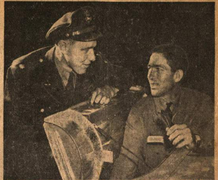
Maj. Alvin J. Mueller, four times decorated for his air exploits in the Pacific area, views construction in Consolidated Aircraft Corporation's plant here of a counterpart of one of the bombers he flew in Australia. The Consolidated employe working in the escape hatch is R. L. Jones.
