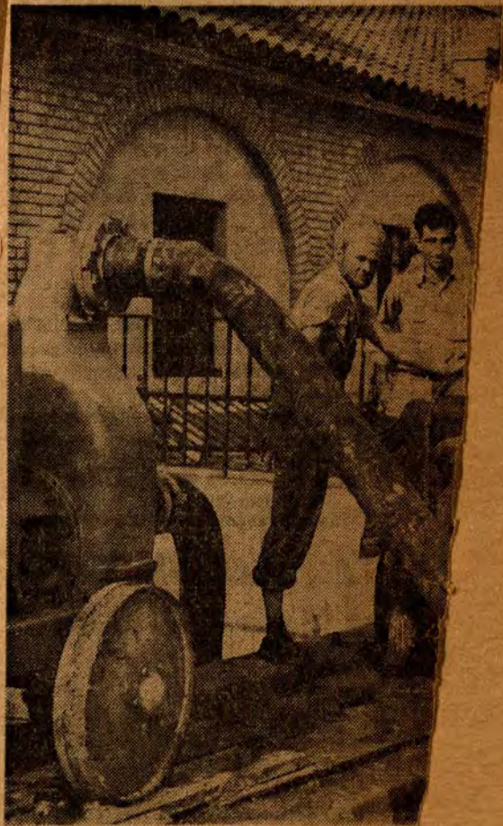
FLOOD PUMP AT WORK —Flood filter building Wednesday by motor service to the city. At left is Harry Carter, who had been on duty 24
