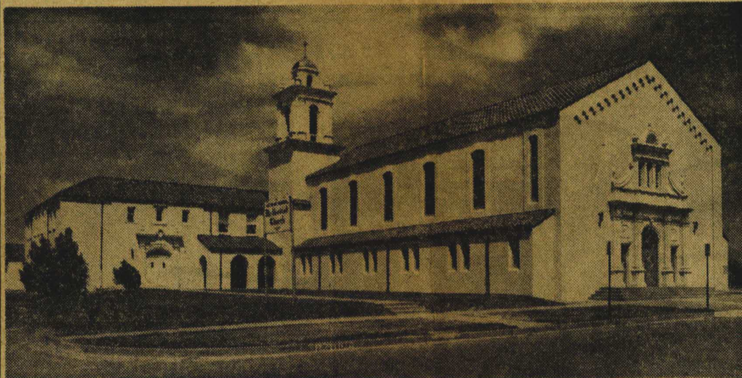
DREAM REALIZED —The new $200,000 Matthews Memorial Methodist Church will be formally opened Sunday at 10:50 a. m., with a former pastor, Rev. T. Edgar Neal of Amarillo, preaching the sermon.
