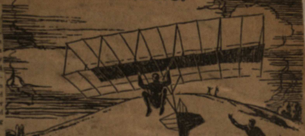
OCTAVE CHANUTE'S BEST GLIDER WAS A BIPLANE WITH WHICH HE MADE A GLIDE OF 360 FEET.
