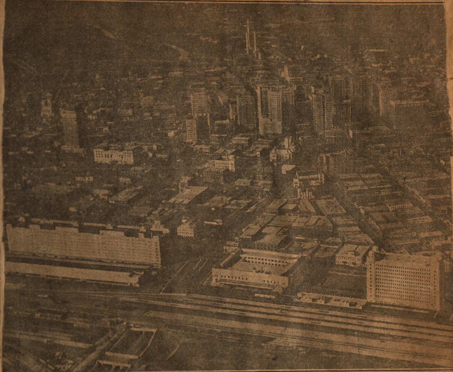
Fort Worth's skyline—as seen from an airplane. This latest photograph of the downtown area was taken from a point just south of the Texas and Pacific Railroad tracks and shows, in the foreground, the T. & P. freight depot, the Jennings Avenue underpass, the postoffice and the T. & P. passenger station. The picture was taken from the plane of Airport Manager W. G. Fuller, piloted by Homer Traux.
