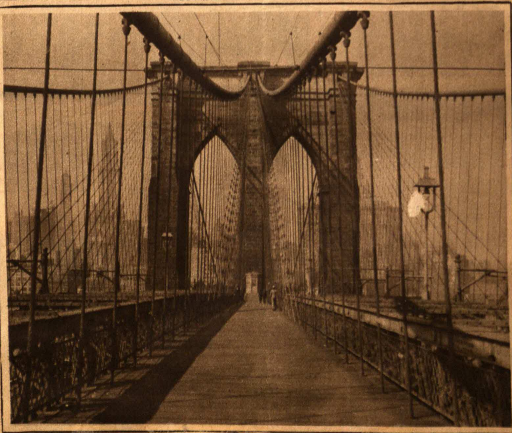
A VISTA OF CABLES. This interesting picture presents a view of the pedestrians' walk of the Brooklyn Suspension Bridge.
