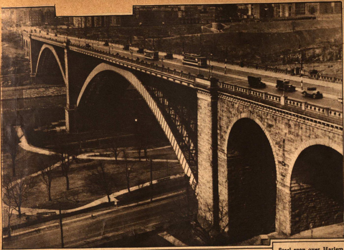
Steel span over Harlem River.
