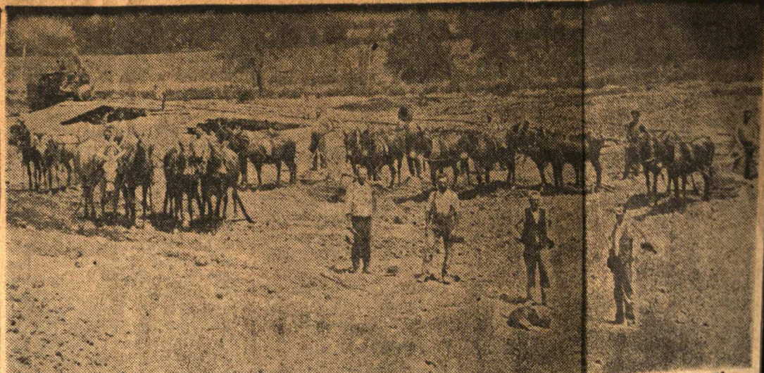
TAKES SECOND PRIZE—This photograph, showing workmen excavating for the packing houses about 1901, was submitted by J. R. Miller, 2810 Clinton, and took second place in the Star-Telegram's Old Photo Contest.
