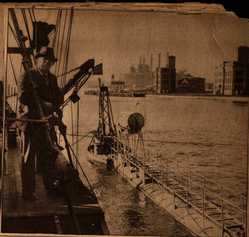
A VETERAN SUBMARINE INVENTOR DIRECTS OPERATIONS IN THE EAST RIVER: SIMON LAKE, From the Deck of the Mother Ship Lillian, Demonstrates His Latest Invention, the Submarine Salvage Craft Lakso, Designed for Tidal Operations Under Which Or- dinary Diving Methods Would Be Impossible, as It Raises Coal From a Sunken Barge Off North Brother Island.
