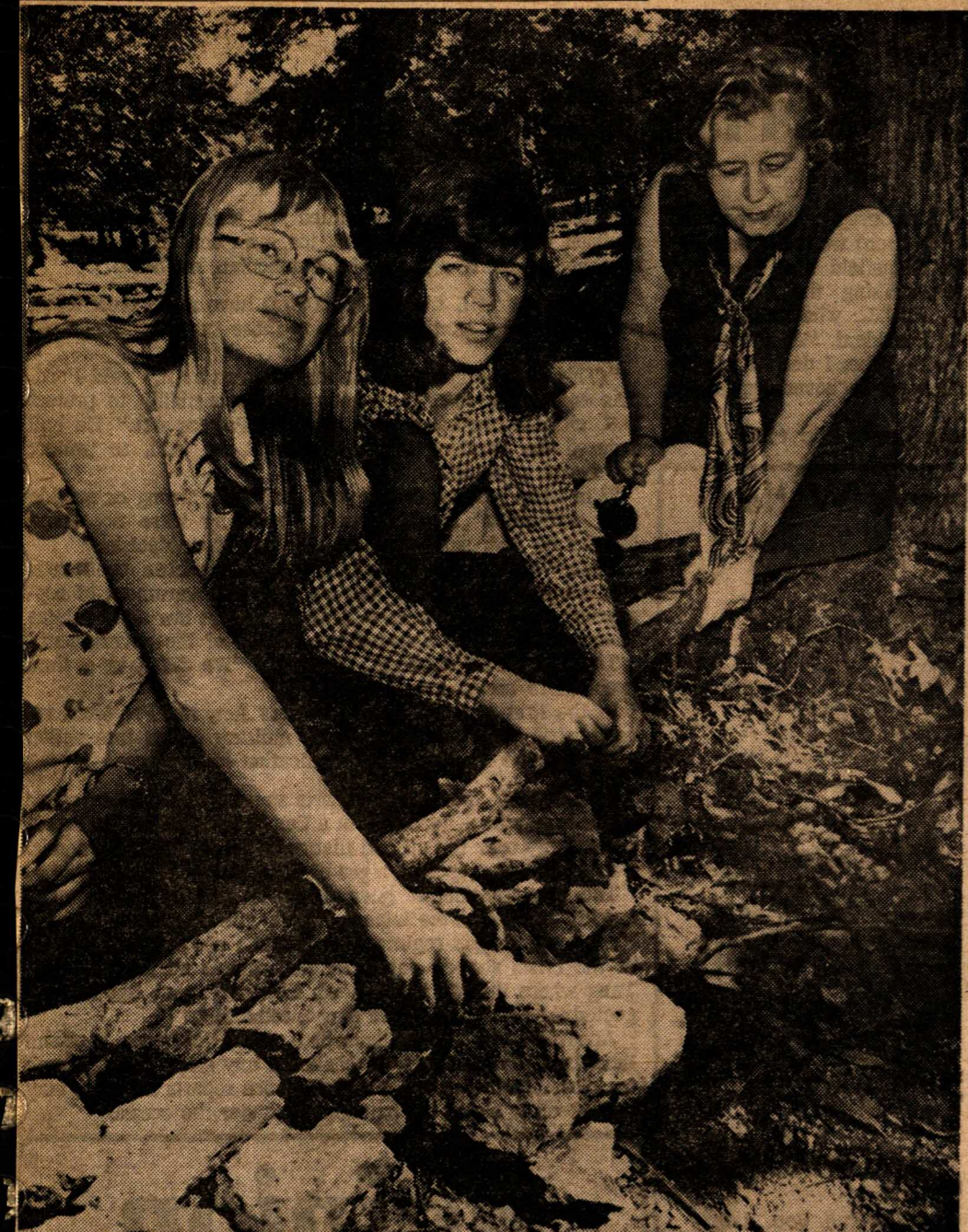
Melba Croan, right, shows Alice Amsden, left, and Deanne Croan how to build a check dam to prevent erosion by stacking rocks around an exposed root. Mrs. Croan is ecological training director for the Texas Section of the American Camping Assn. —Press Staff Photo by Gene Gordon.
