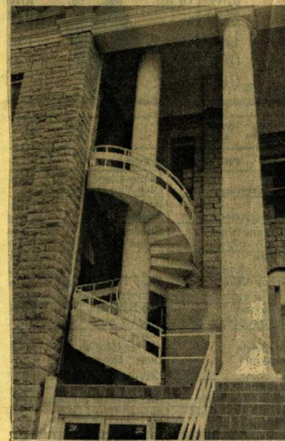
Star-Telegram Photo RESTORATION... at Texas Wesleyan
