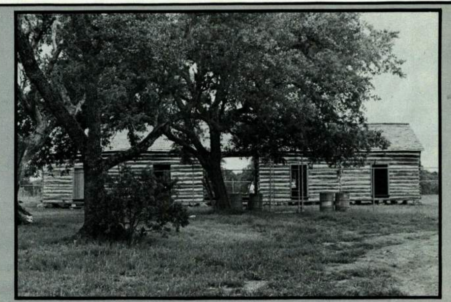
CLAIBORNE KYLE LOG HOUSE, Kyle, Hays County, designated as a Recorded Texas Historic Landmark. Constructed of hand-hewn cedar logs, this four-pen dog trot home dates to the mid-19th century. Col. John Claiborne Kyle and his wife, Lucy, built the vernacular structure. A prominent pioneer family, the Kyles had five sons serve in the Confederate army, including Capt. Ferg Kyle, for whom the town of Kyle was named.
