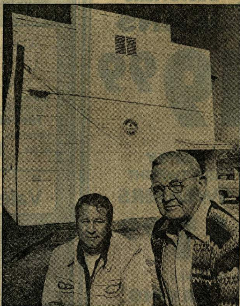
THE SMITHVILLE MASONIC LODGE, fronted by Ray Tomes, left, and Fred McCullar, is looking for an owner.
