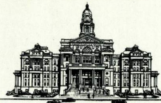
TARRANT COUNTY COURT HOUSE FORT WORTH, TEXAS
