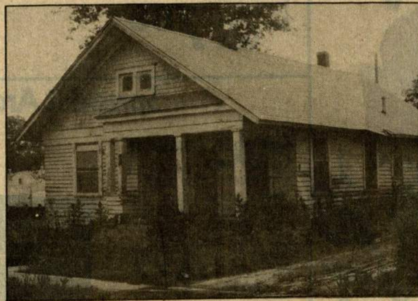
The house at 1705 Fifth Ave. before renovation
