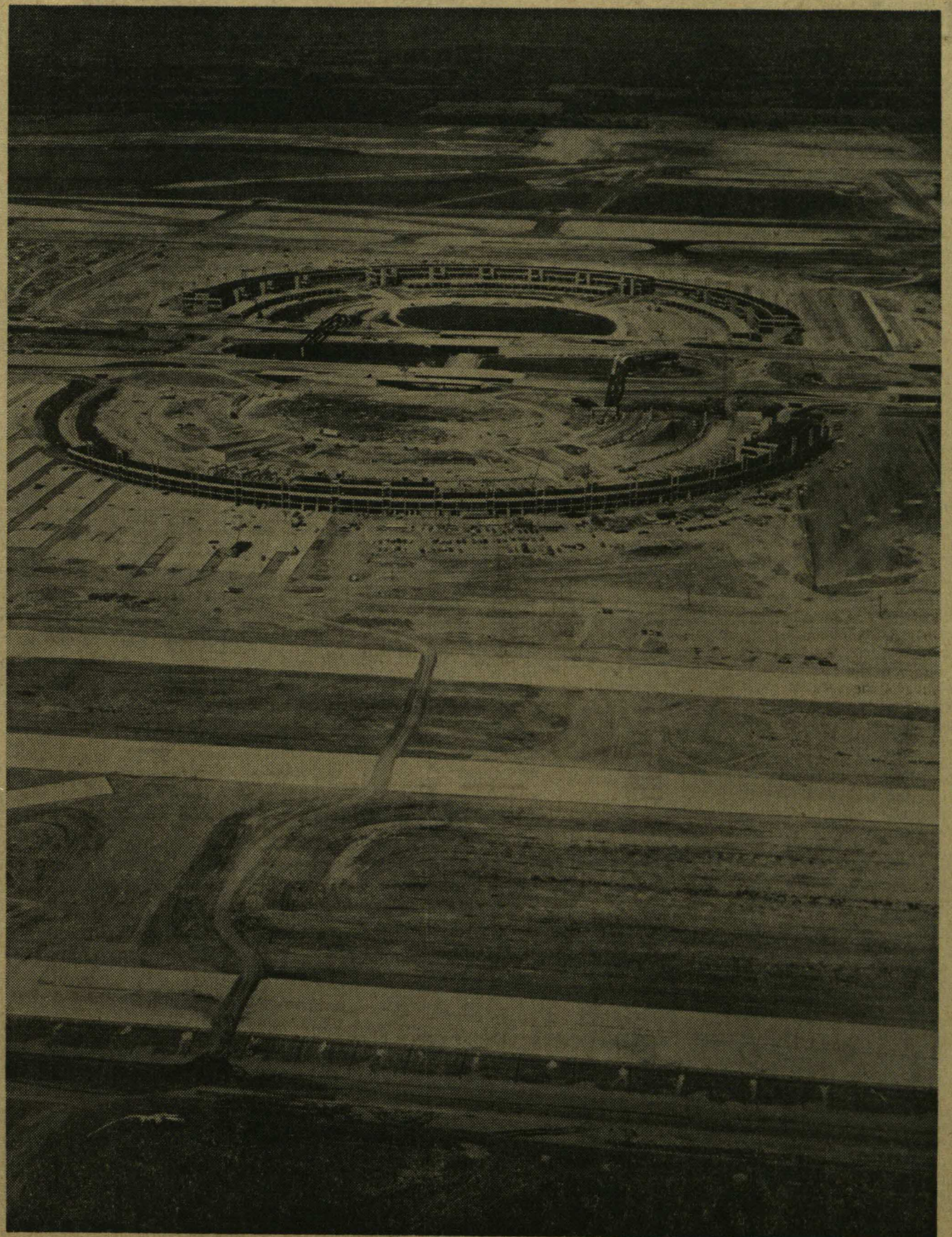
PLANE SIDE — This view of Dallas-Fort Worth airport, looking west, shows one north-south runway and two taxiways nearing completion (at bottom). Planes will load and unload on aprons outside the semi-circular terminals. Automobiles will park within
