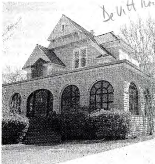
The circa 1902 Victorian-style house at 3325 W. Seventh St. is in the way of development. STAR-TELEGRAM/RODGER MALIKIAN
