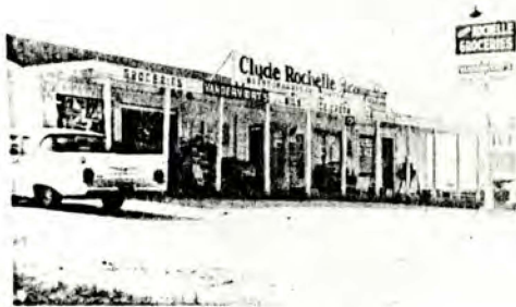
Clyde Rochelle Grocery Building
