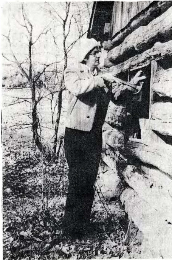
TAGGING UP- Ms. Barker nails home metal tags marking the location of each log.
