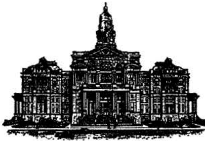
Tarrant County 1895 Courthouse
