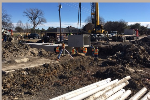
Precinct 3 Maintenance Crew setting concrete box culverts on Willow Springs Road.
