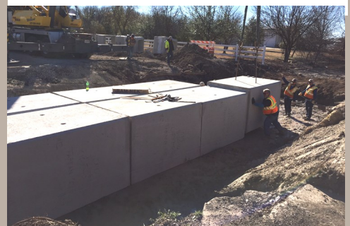
Precinct 3 Maintenance Crew setting concrete box culverts on Willow Springs Road.
