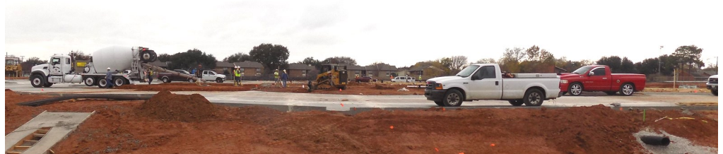
Construction in progress for the new JPS Medical Home Northeast Tarrant
