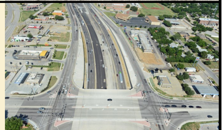
(Photo shows new Main St. bridge in Euless taken on May 22, 2018)
