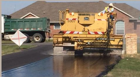
Pictured above: Improvements made to Haslet Heights and Country Ridge Estates using the chip seal process. During this process, liquid asphalt is applied to the surface and is followed by a layer of crushed gravel which is embedded by the pneumatic roller. After a few days, the excess rock is swept up.
