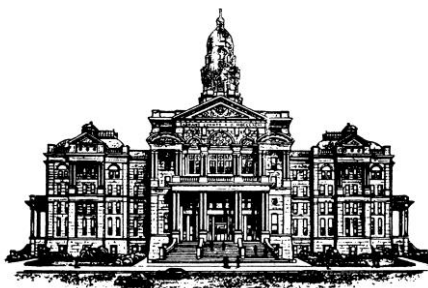
Tarrant County 1895 Courthouse
