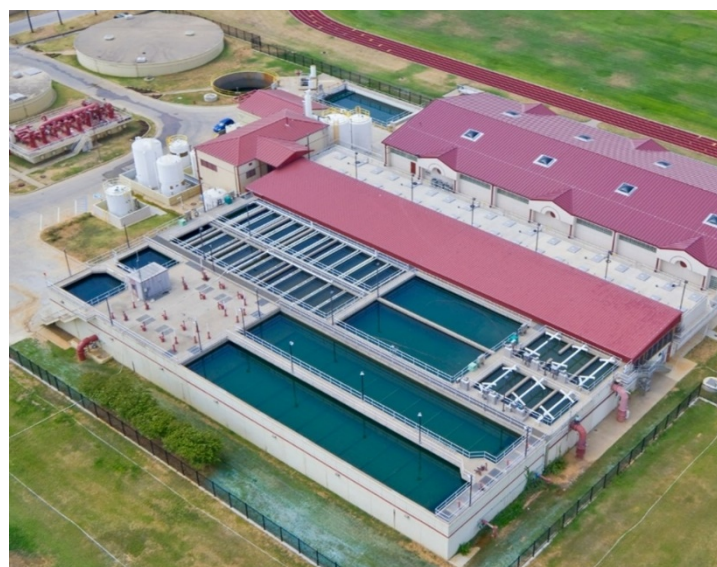
Bud Ervin Water Treatment Plant
