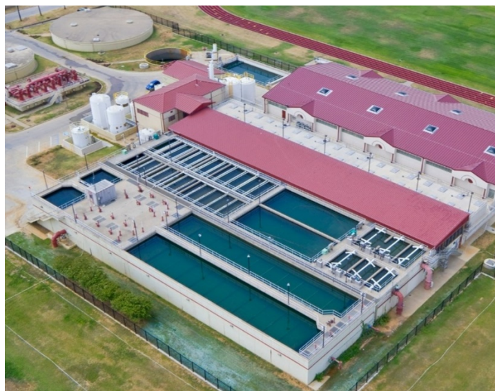
Bud Ervin Water Treatment Plant
