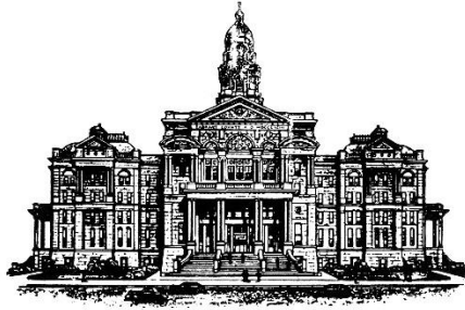
Tarrant County 1895 Courthouse
