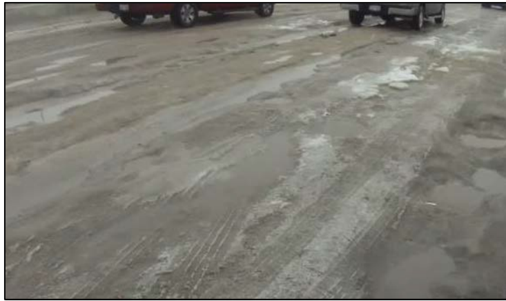
Figure 90: “Cobblestone ice” on North Texas Roads 132
